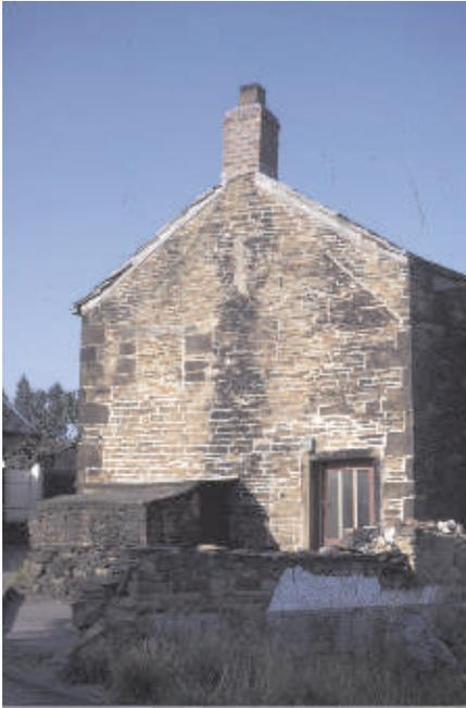
**The gable-end of this old weaver's cottage in Radcliffe Street, Skelmanthorpe shows how the roof of the house was raised so that the handloom could be fitted with a Jacquard to operate effectively.**
